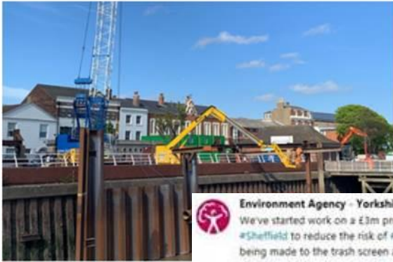
Work to install the new flood defences in Nelson Street
