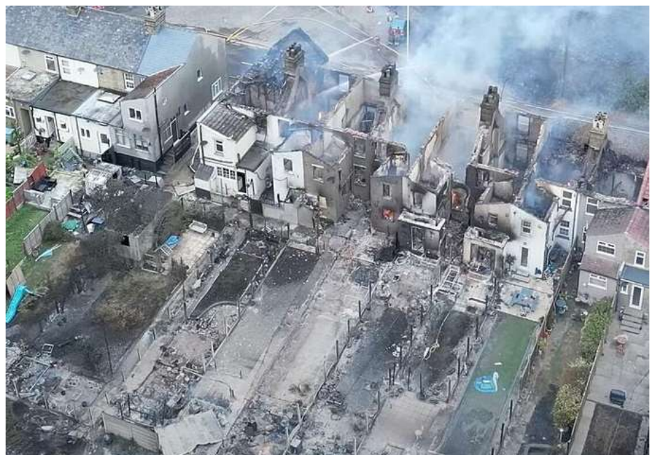
■ The row of houses destroyed in Wellington, during the 2022 heatwave
